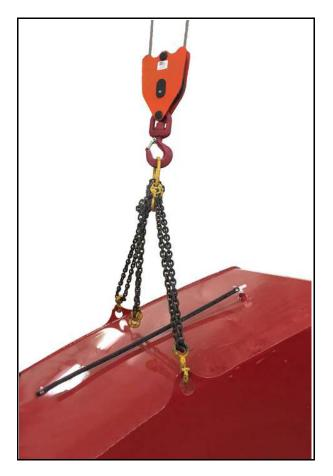
1.Connect an appropriate lifting device to the top lift points on the tank.
