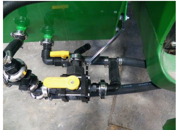
Figure 2: Right-hand tank plumbing assembly
