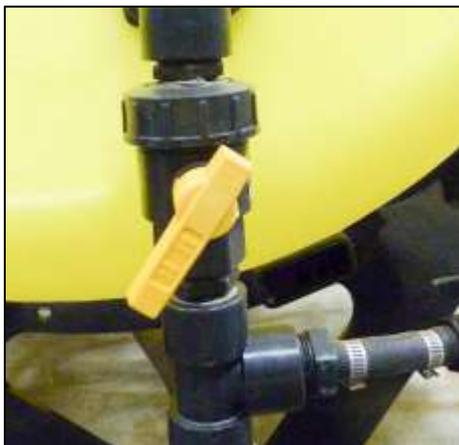
Figure 15: Control valve in normal working position
